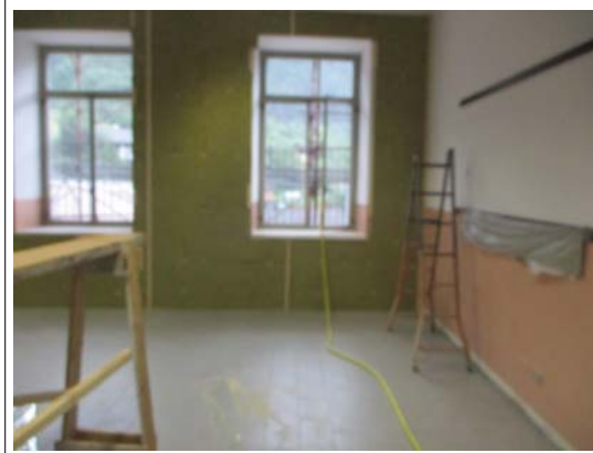
Isolamento parete aula. by Arch. Sergio Ghirardelli (DL)
