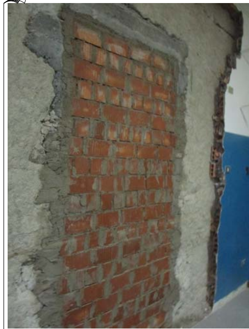
Riempimento nicchia al piano terra. by Arch. Sergio Ghirardelli (DL)
