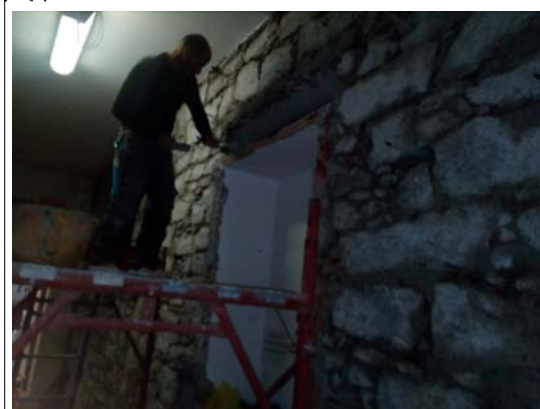
Ripristino muratura sconnessa by Arch. Sergio Ghirardelli (DL)
