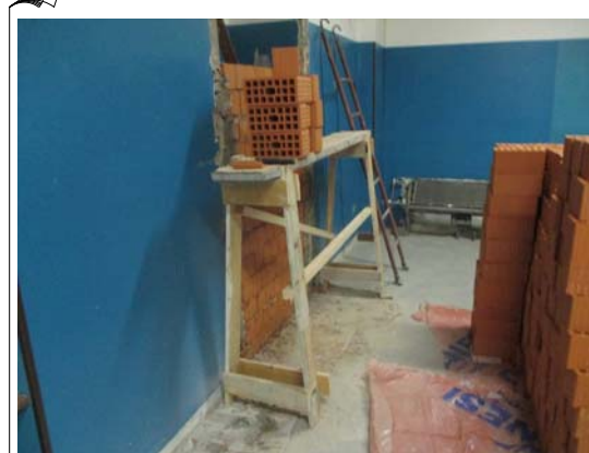
Riempimento nicchia piano terra. by Arch. Sergio Ghirardelli (DL)
