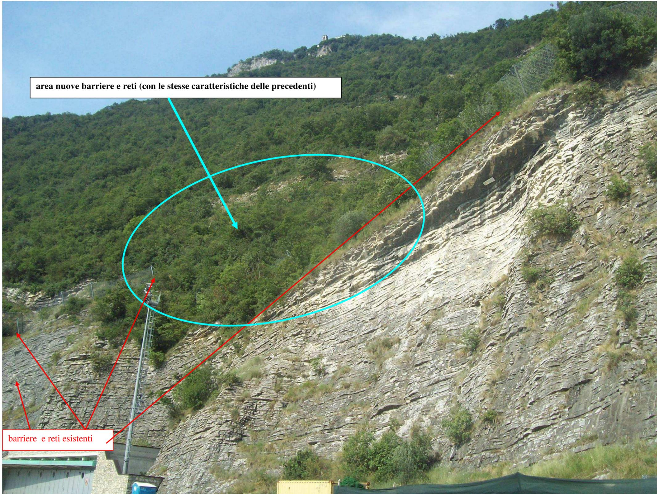
ESEMPI BARRIERE PARAMASSI CON ASSORBIMENTO ENERGIA (MEL) 2000 KJ
